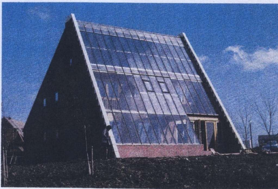
View of the south side of the house, showing the double storey height conservatory and the solar panels above.
