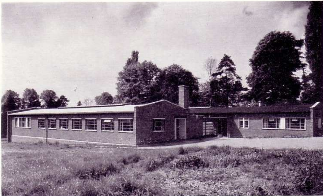
Engineering and Metallurgy Laboratories
