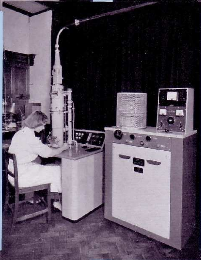
ABOVE Geiger counter spectrometer for liquid metal studies
